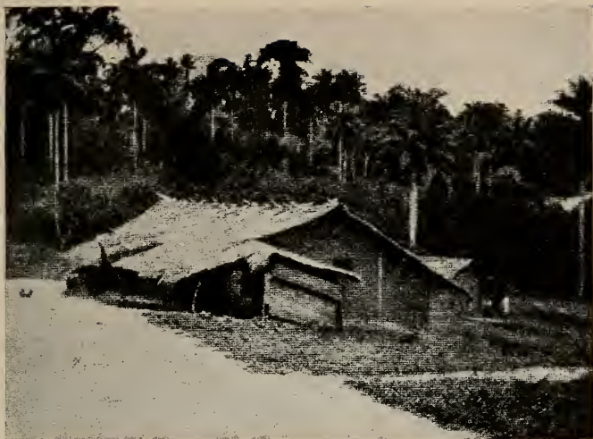
COURT HOUSE AT IKOTOBONG
