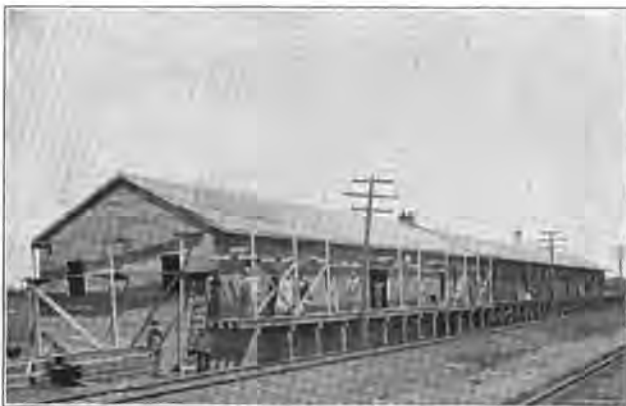
ZION CITY FREIGHT HOUSE.
