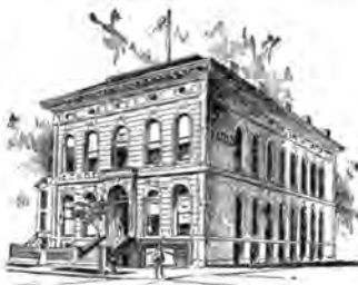
ZION COLLEGE BUILDING.
