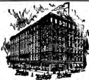
ZION HOME, Michigan Avenue and Twelfth Street, CHICAGO.
