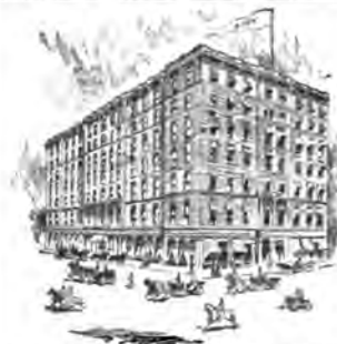
ZION HOME, Michigan Avenue and Twelfth Street.
