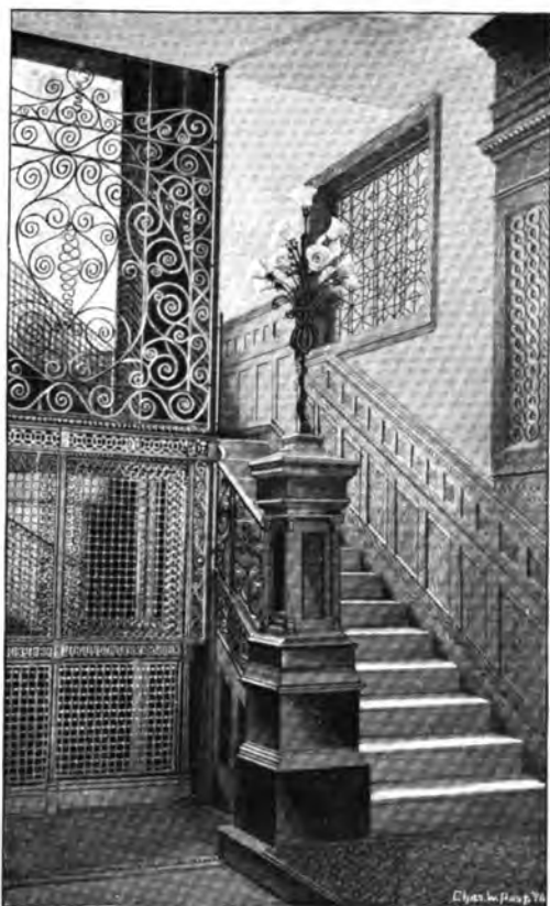
Passenger Elevator and Staircase.
