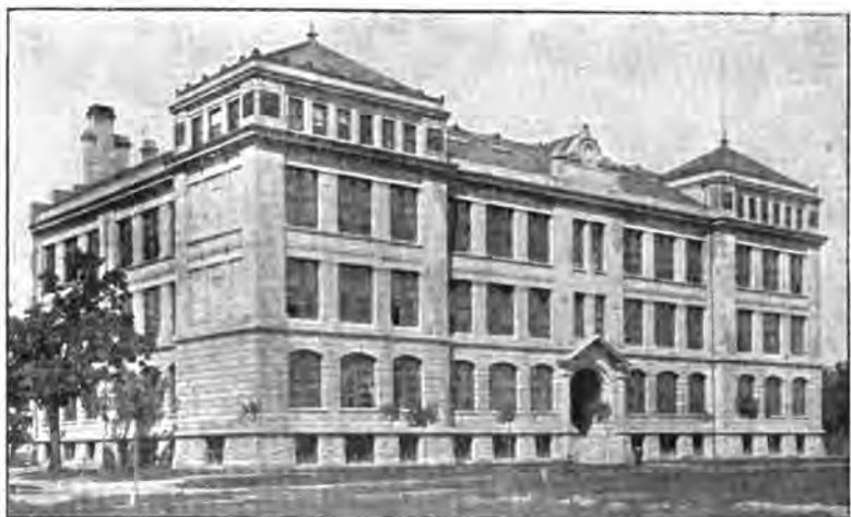
EAST WING ZION EDUCATIONAL BUILDING.
