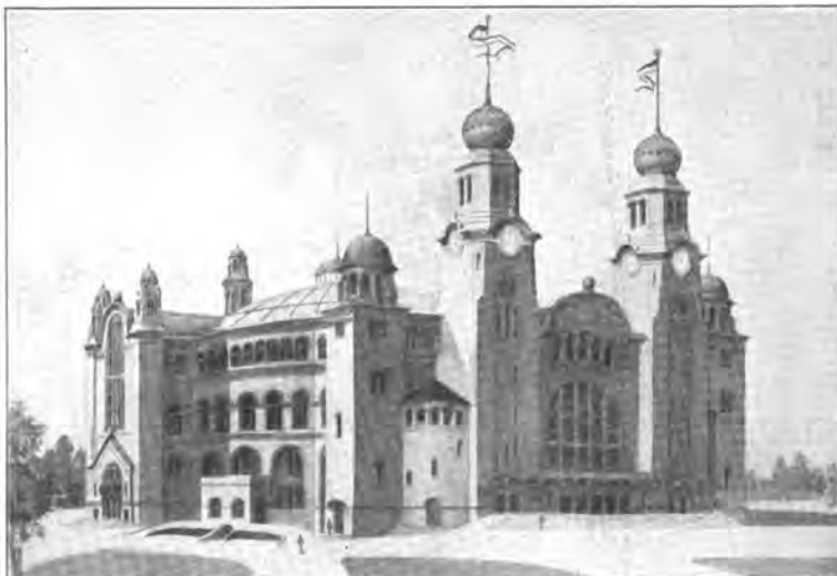
SHILOAH TABERNALE AS PLANNED, Now in Course of Construction, Shiloh Park, Zion City, Illinois. To seat 16,000 people.
